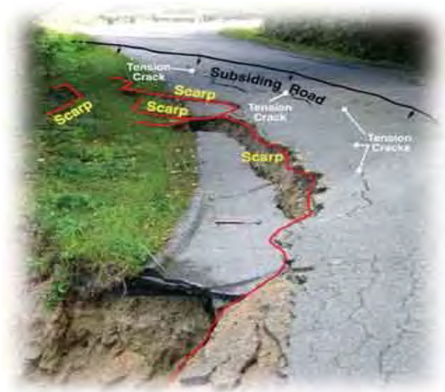
This picture shows landslide damage to a roadbed similar to that found in flash flood events in Richland County. 74
