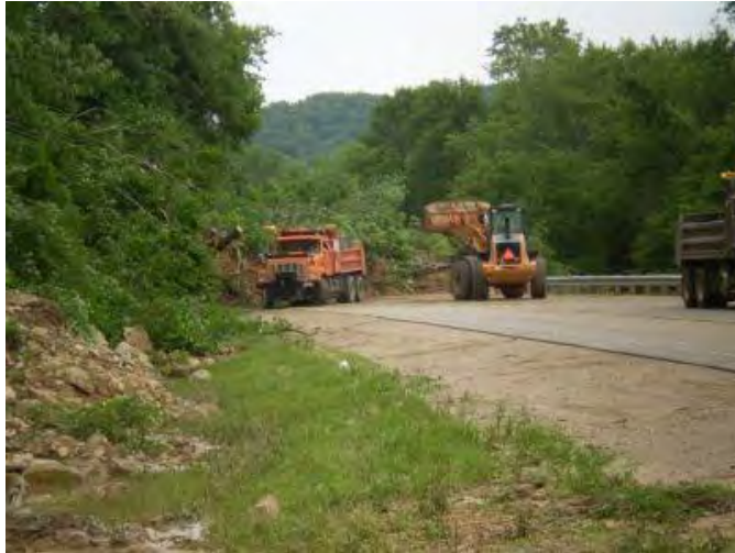
Highway 61 landslide clearing near Boscobel, WI.
