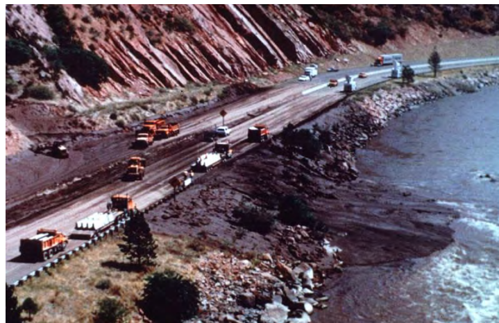
Landslide from fire damage in CO 75
